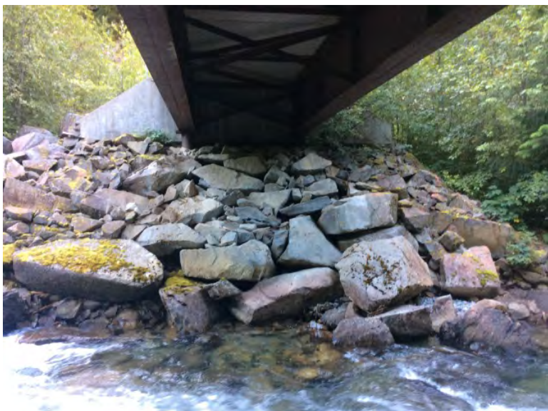
Left Bank Abutment when facing downstream
