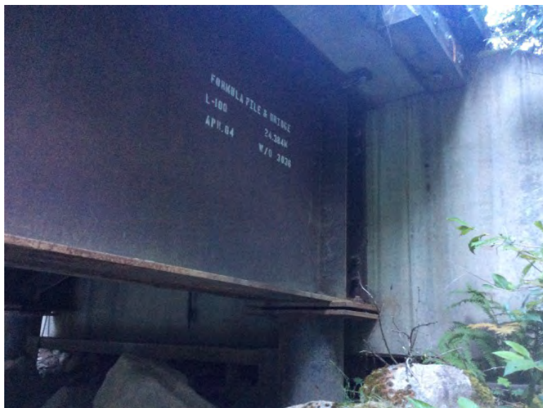
Right Bank Abutment when facing downstream
