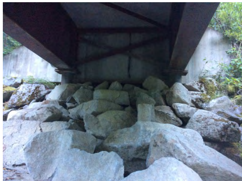
Right Bank Abutment when facing downstream
